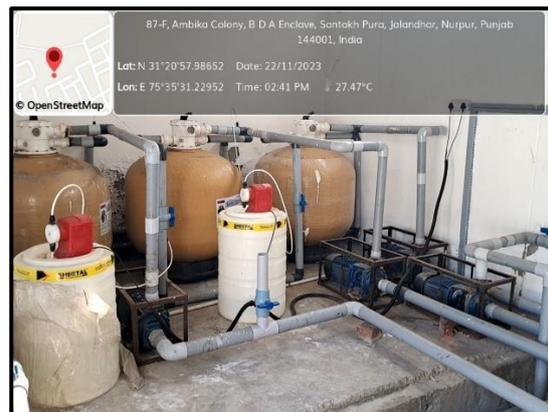
**Figure 3: Sand Filtration Plant for recycling of water**
